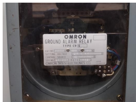
Ground over voltage relay
