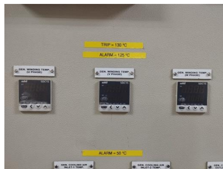
Temperature indicator for stator coils
